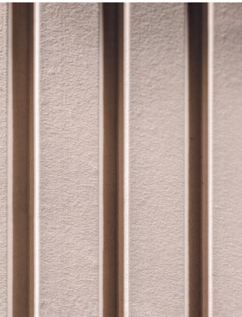
Chamotte combustion chamber lining with grooves:
