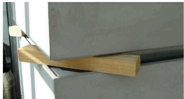
Im. 3: Wood pieces as supports
