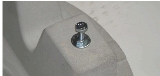
Illustration 4: Bolt in base plate
